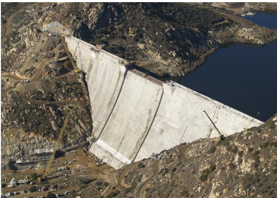
Aerial view of the San Vicente Dam downstream slope after completion of the dam raise using RCC, giving an appearance of a concrete staircase.
